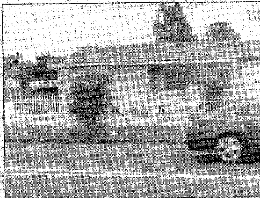
Neighbouring dwelling at 45 Edensor Road.
